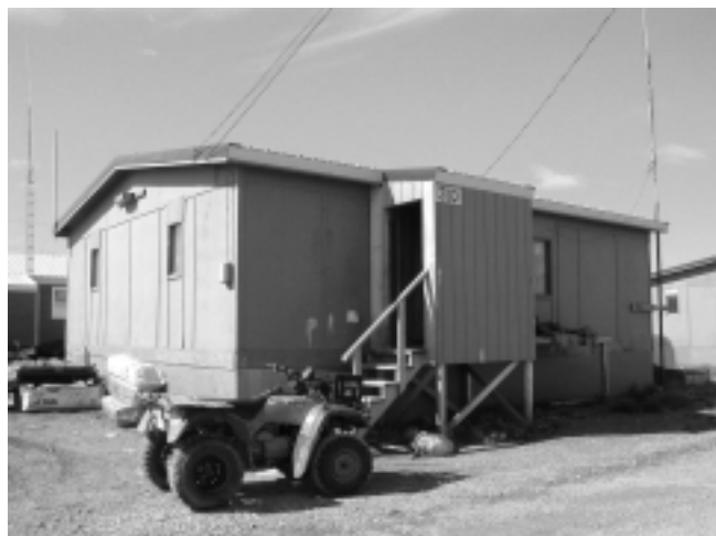
Figure 2: A typical house in Arviat, Nunavut
