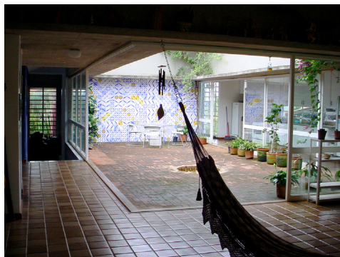
Fig. 5. (a) NS-axis, atrium and kitchen – reinforced concrete allows elimination of traditional peripheric columns, thus stressing spatial continuity; (b) kitchen (left), living and doors to veranda (right).
